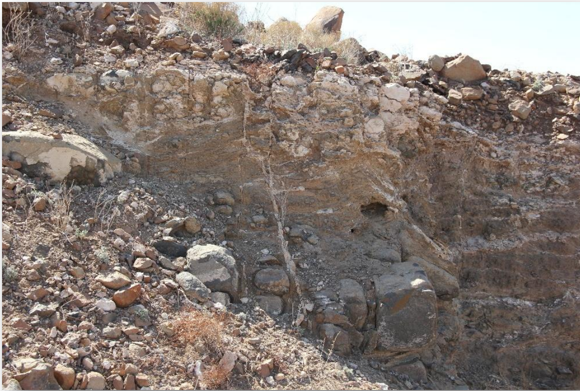
Figure 14. Caliche coatings and associated calcite filled fractures extending down into weathered dolerite, Railroad Dike, N.M.
